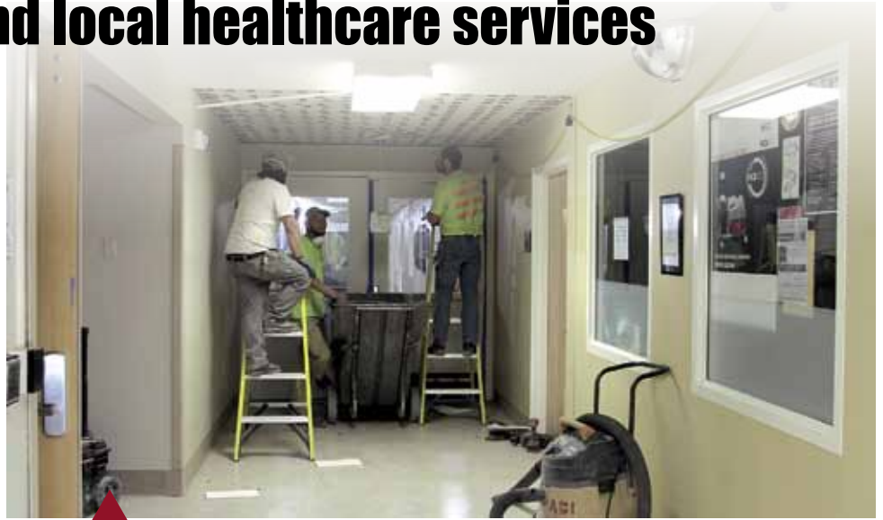
Renovation continues on the area of the hospital that will house the proposed Outpatient Procedure Center
