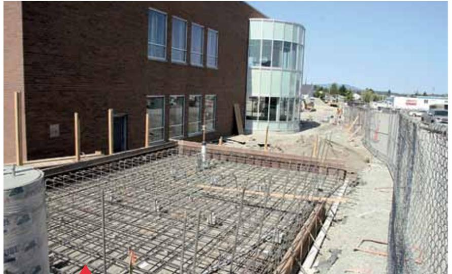
*In early September, work moved to the east and north sides of the Medical Arts Pavilion. The concrete formwork will support the oxygen tank. There will be a significant demand for oxygen to operate the hyperbaric chambers in Wound Care as well as supplemental oxygen use in Cancer Care.*
