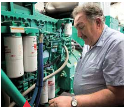
Mel Larsen checks fuel filters on the hospital's emergency generator.
